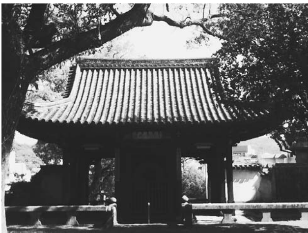
back side of the inner gate
